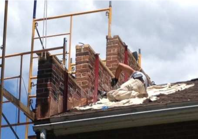
Workman from Turner Construction attaching copper flashing to back of façade at Priestley Chapel. Note the steel re-enforcing bars.
