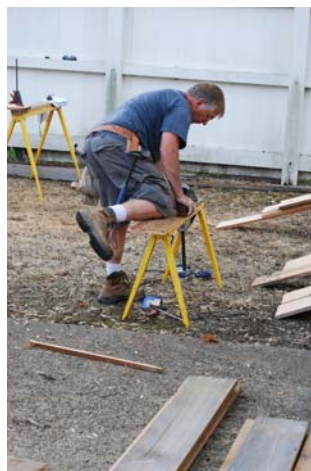
Frank Stroik uses a 19 th century plane as he works on a piece of siding.
